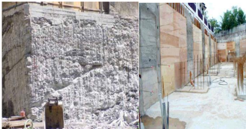
Smoothing the rough surface by removing undulations and sharp protrusions and fixing the plywood to make the surface smooth
