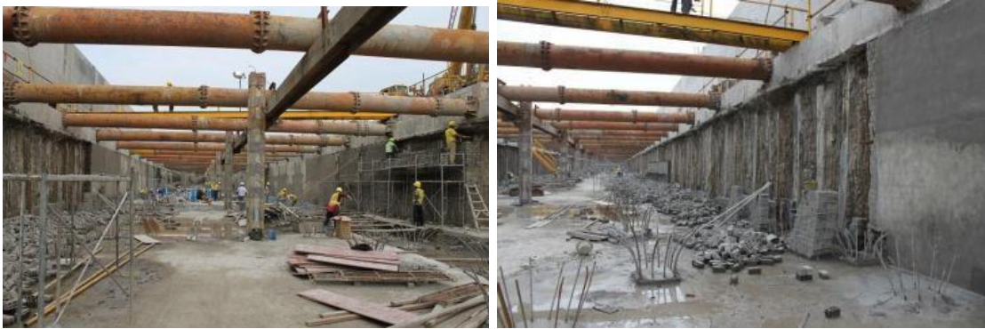
Smoothing the surface using masonry or cement mortar
