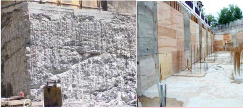
Smoothing the rough surface by removing undulations and sharp protrusions and fixing the plywood to make the surface smooth
