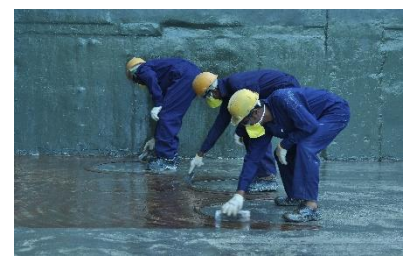
Application of epoxy primer putty
