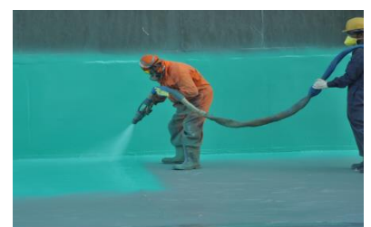
Application of Fosroc's Polyurea WPE
