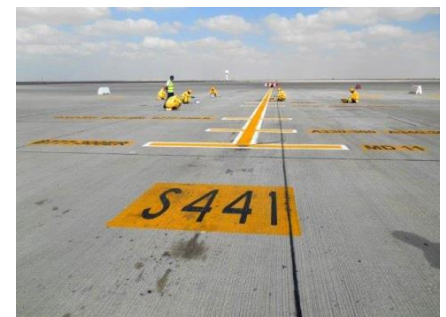
Colpor 200 applied on the Taxiway
