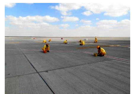
Colpor 200 applied on the Apron/Runway
