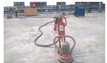
Grinding surface preparation
