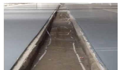
Finish floor Nitoflor SL3000 UT application
