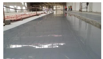
Nitoflor SL3000 UT 4mm thick application
