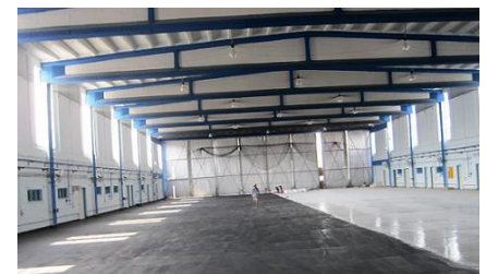
Application of ESD topping in progress after undercoat
