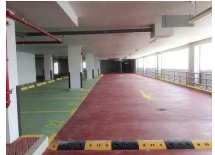
Trafficguard UR250 indoor applied
