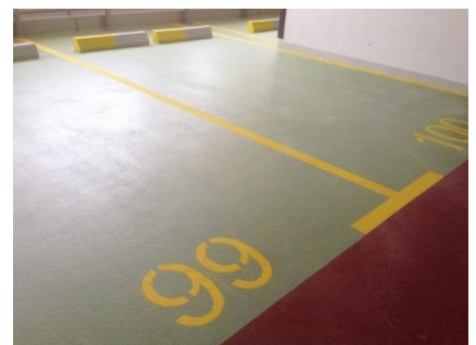
Trafficguard UR250 indoor applied
