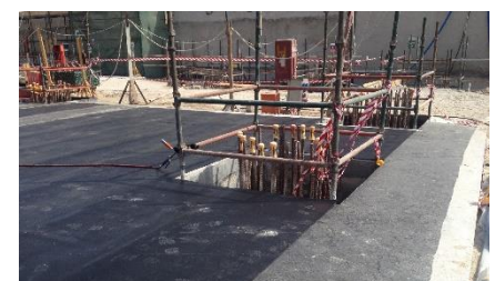
Pile cap Details for PROOFEX TORCHSEAL 4S
