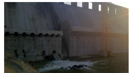
Valley side view of the dam
