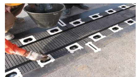
Colpor 200 sealant application
