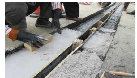
Bridge Transition Strip surface preparation by Nitomortar S
