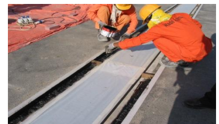
Nitomortar TS application
