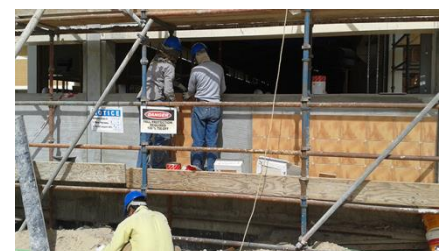
Tile fix using Nitotile 489
