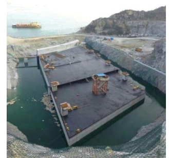
Completed Single Precast Section at Qi Wan precast dock
