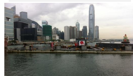
Precast immersed tube being towed into position at the Victoria Harbour
