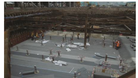
Proofex Engage applied on-site
