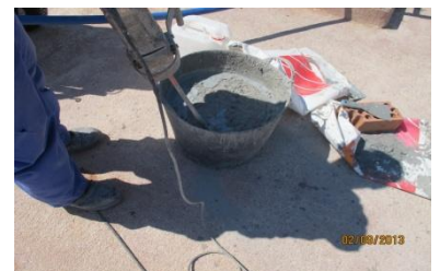
Mixing of Nitocote CM660
