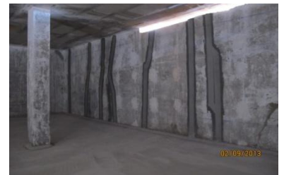
Preparation and repair of the support with Renderoc SFBD
