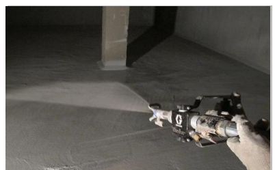
Spray of Nitocote CM660
