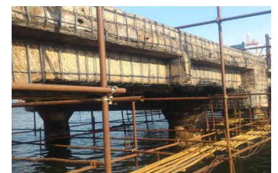
Scaffolding suspended from the top using T-joint connections
