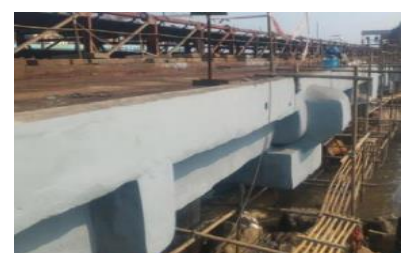
A reinstated structural members finished with Nitocote PE 135
