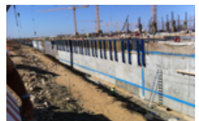
View after Fixing S/Cast PVC & Casting
