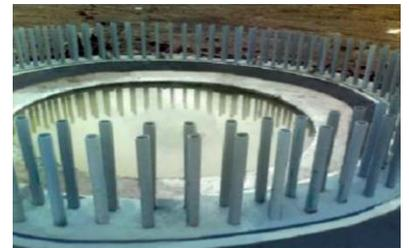
Anchor bolt fixing
