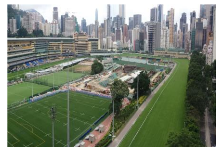
Excavation from northeast of the recreation ground
