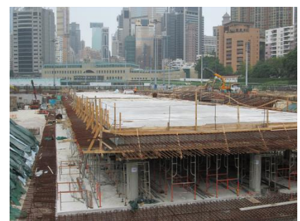
Section of top slab of the stormwater tank completed
