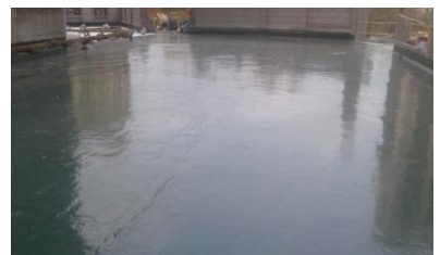
Nitoproof 600 PF after application
