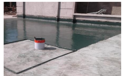
Application of Nitoproof 600 PF
