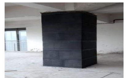
CFRP wrapped RCC Columns for enhanced load capacity
