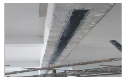
Flexural Strengthening of RCC beams with Nitoplate CPS
