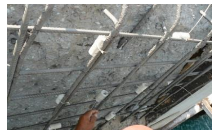
Recasting along the waterline
