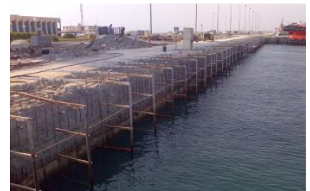
Installation of Galvashield
