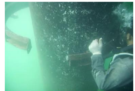
Divers installing Fosroc Marine Jackets
