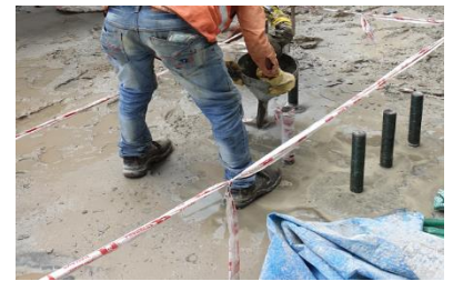
Application of grout
