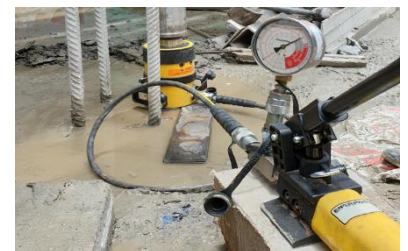
Fixing pull out testing equipment
