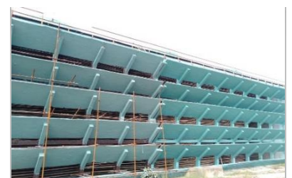
Dekguard E2000 for IDCT Cooling towers after repairs
