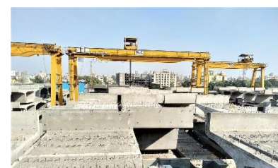
Metro rail casting yard
