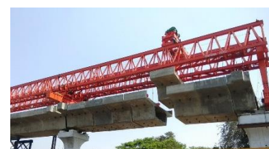
Launching 1st girder for Line 2
