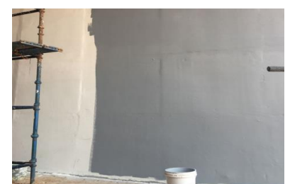
Box Culvert coated with Dekguard E 2000 RAL 7001 Silver Grey
