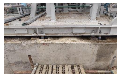
Area to be grouted
